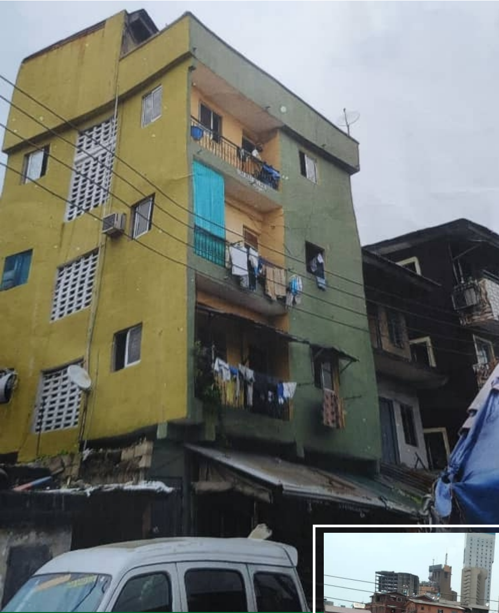
Five- storey building that collapsed at No 63, Massey Street, Ita-Faaji, Lagos Island.
