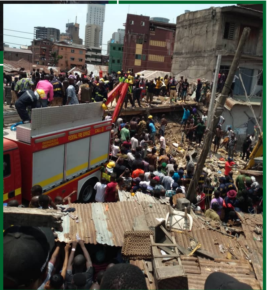
Rescue operation after the building collapsed.
